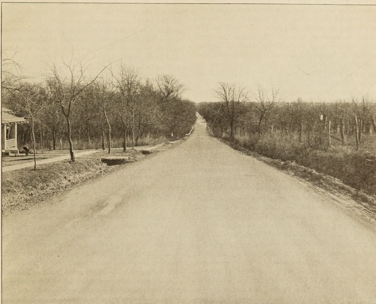
OLD GRAVEL ROAD SURFACE TREATED WITH AN 80 PER CENT ASPHALTIC ROAD OIL. PHOTOGRAPH MADE TWO YEARS AFTER TREATMENT.
